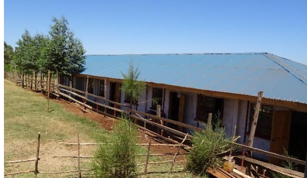
| 4 of the new classrooms next to the sports field
